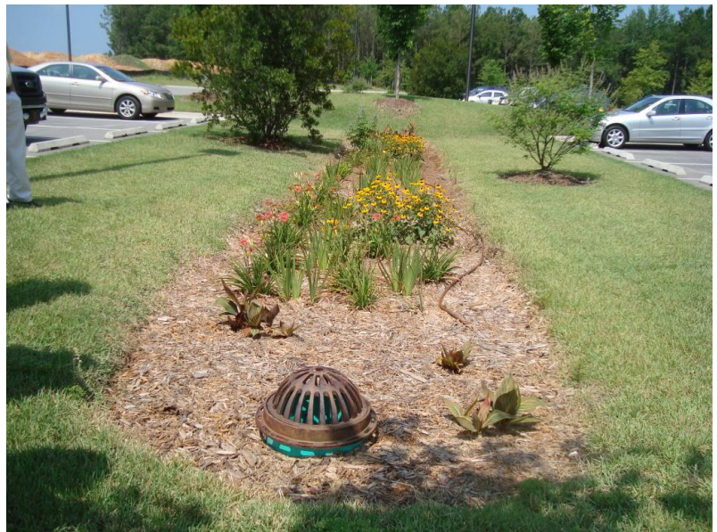
Figure 11: A parking lot with flush curbs draining to a trench in a depressed landscaped area.
