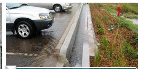
1 Level Spreaders dissipate stormwater runoff energy to protect from erosion
