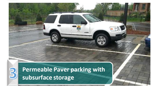
3 Permeable Paver parking with subsurface storage
