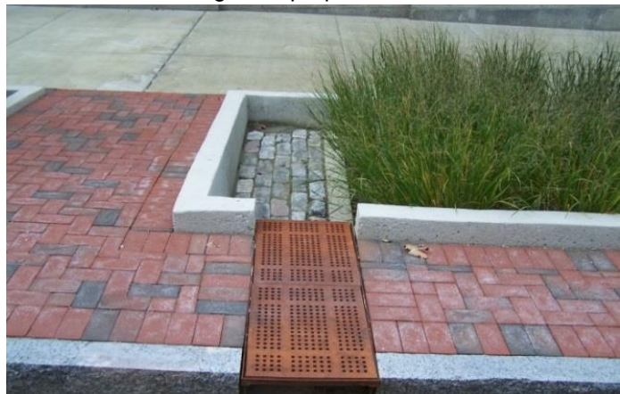
Figure 19: Example of sidewalk trench drain.
