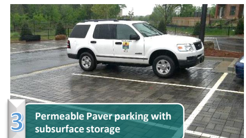
3 Permeable Paver parking with subsurface storage
