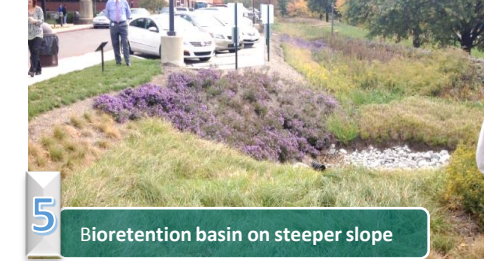
5 Bioretention basin on steeper slope
