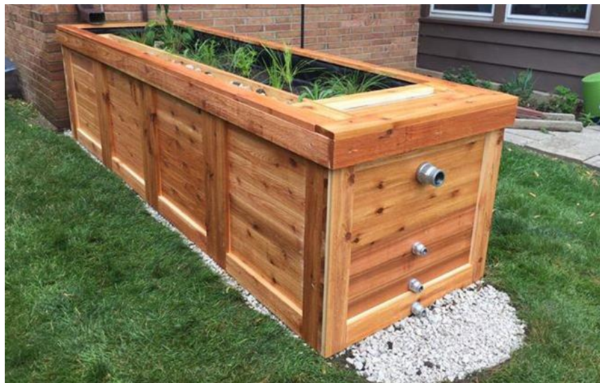
Figure 24: Example of a downspout planter draining a roof leader.
