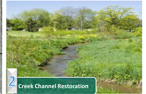
2 Creek Channel Restoration
