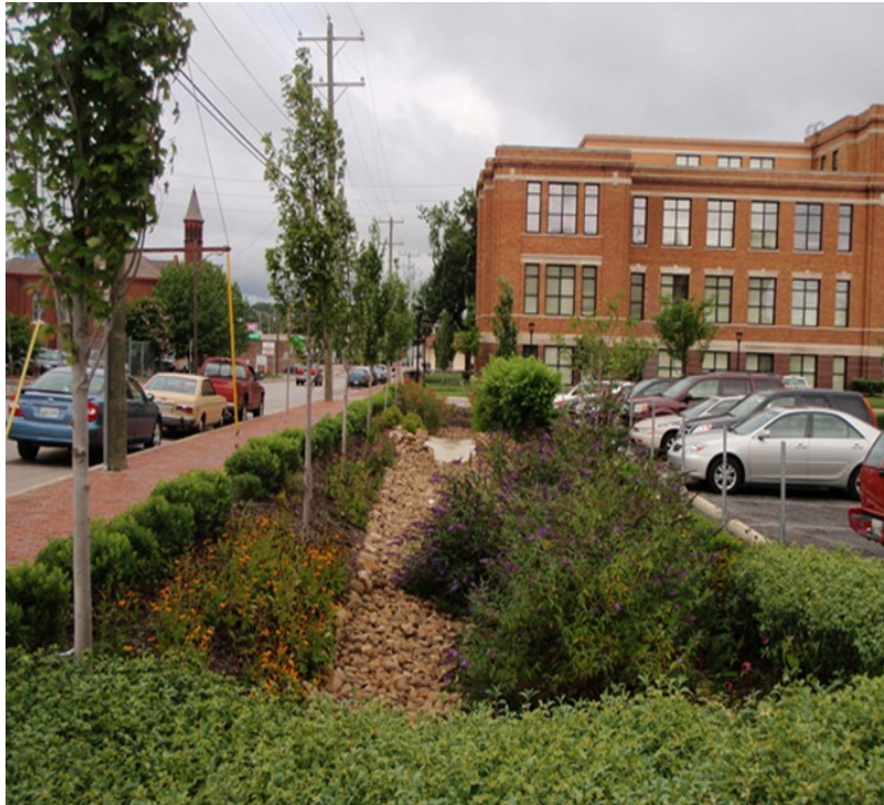
Figure 5: Properly maintained bioretention area.
