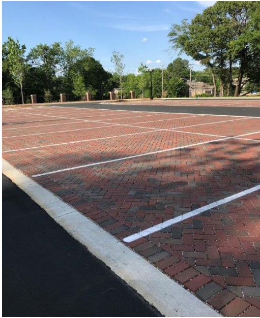
Figure 10: Permeable Pavers featured at the Gay Street Parking Lot in Auburn, AL
