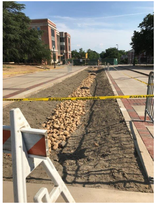
Figure 8: Installation of infiltration area in median in Auburn University.
