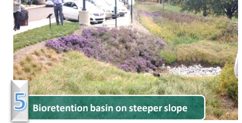
5 Bioretention basin on steeper slope
