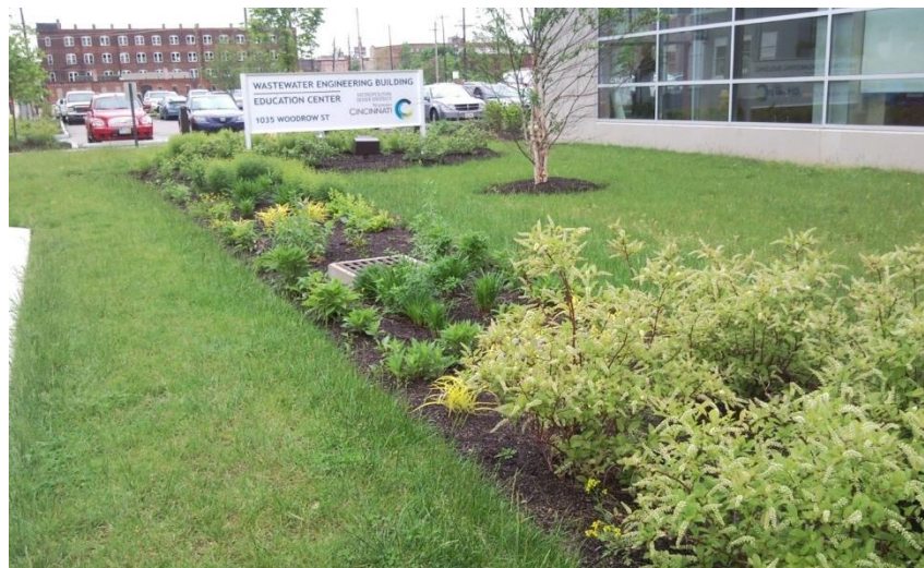
Figure 20: Example of a bioretention area incorporated into landscaping.
