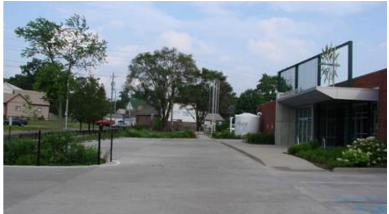
Figure 13: Example of rainwater being harvested and used in conjunction with a bioretention area and pervious concrete.
