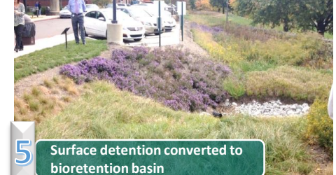
5 Surface detention converted to bioretention basin
