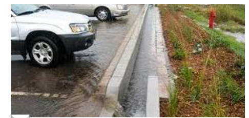
1 Level Spreaders dissipate stormwater runoff energy to protect from erosion
