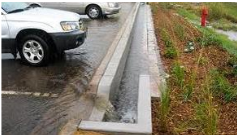
Figure 21: Example of a parking lot draining to a level spreader and bioretention area.
